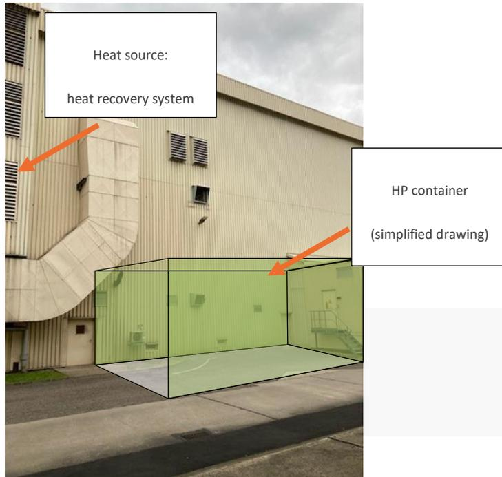
Figure 25: Installation site for HP container solution
